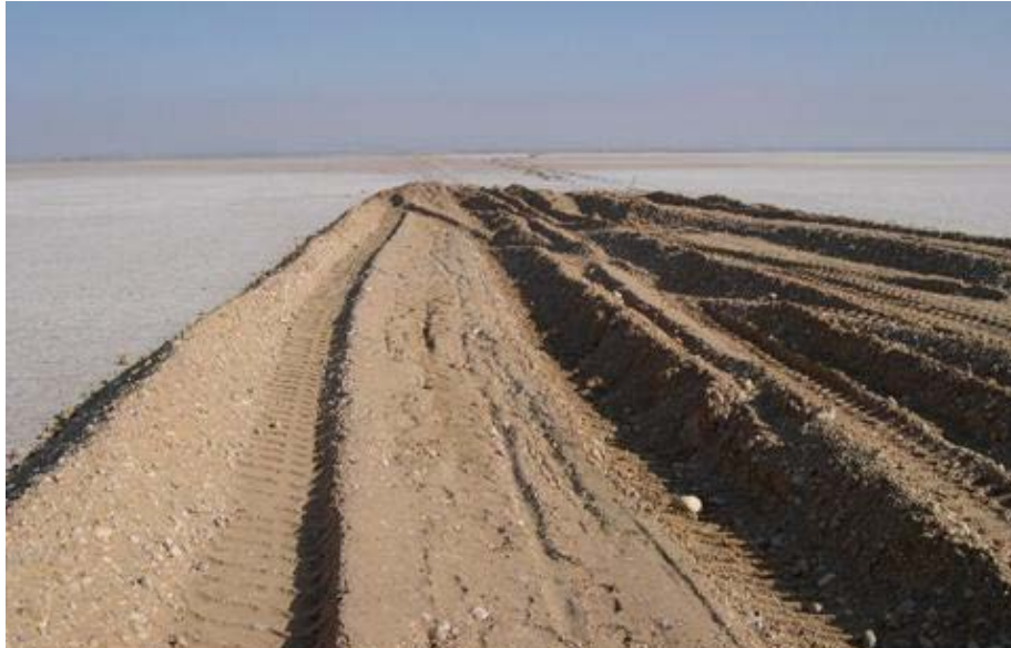
Figure 5: Difficult to construct the first layer embankment
