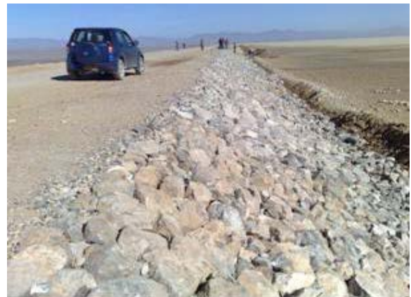
Figure 12: Protection of embankment slopes
